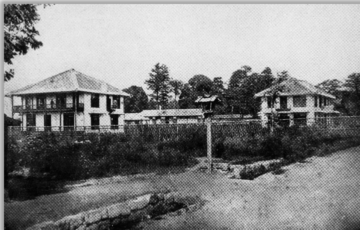
Imadegawa Campus, first buildings (Numbers 1 and 2)
