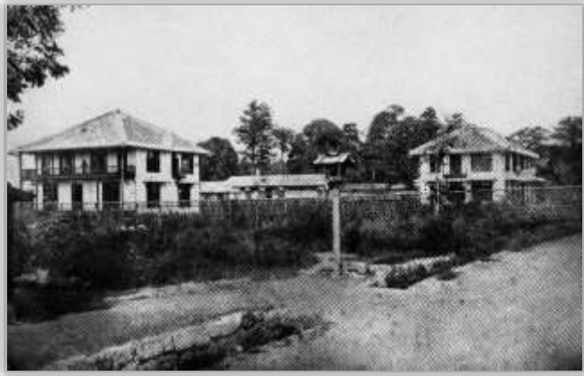
Imadegawa Campus, first buildings (Numbers 1 and 2)
